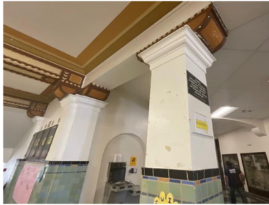
Figure 4: Area B1 – Missing touch-up paint around columns
