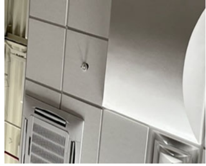
Figure 7: PAC – Band Area – Ceiling tiles have gaps around sprinkler heads
