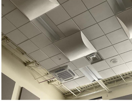
Figure 7: PAC – Band Area – Ceiling tiles have gaps around sprinkler heads
