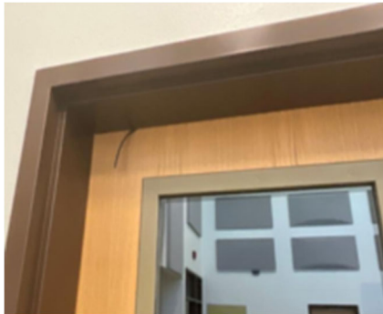
Figure 8: PAC -Orchestra Area – Door seal coming off PG110A Practice Room A. Issue has been corrected.
