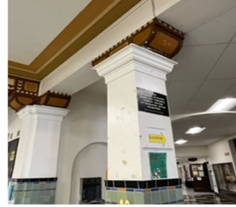
Figure 4: Area B1 – Missing touch-up paint around columns
